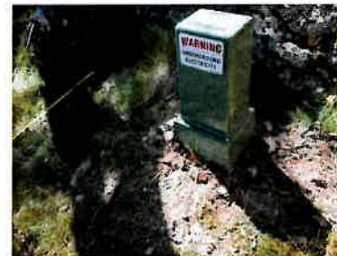
Electricity pillar with work commenced
